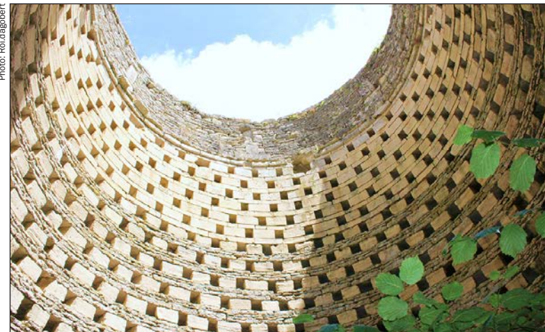
An inside look at the roosts or boulins in this cone-shaped colombier that is still standing in good condition at Rosel near Caen in Calvados
