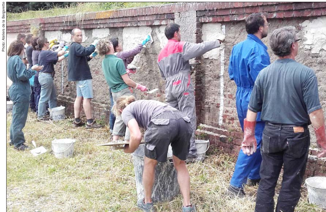
Jan Minne works on pointing with lime mortar and the photo, right, from Ateliers de la Bergerette shows the interest in learning lime rendering methods
