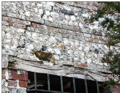
Jan Minne was called in to save this wall where the timber lintel was failing and sinking, meaning all the stonework above was at serious risk of collapse
