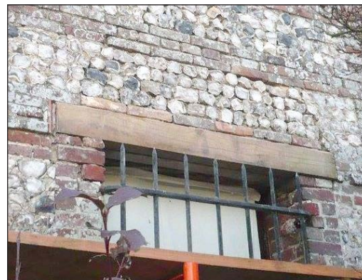
Jan Minne was called in to save this wall where the timber lintel was failing and sinking, meaning all the stonework above was at serious risk of collapse
