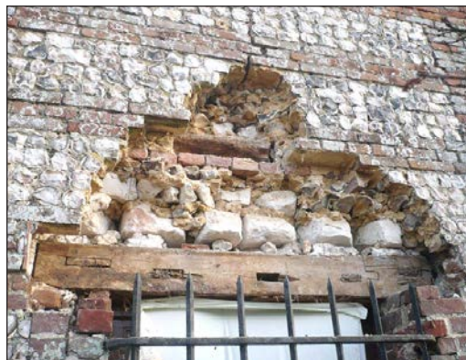
Jan Minne was called in to save this wall where the timber lintel was failing and sinking, meaning all the stonework above was at serious risk of collapse
