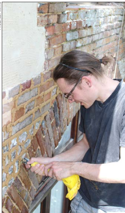
Jan Minne works on pointing with lime mortar and the photo, right, from Ateliers de la Bergerette shows the interest in learning lime rendering methods
